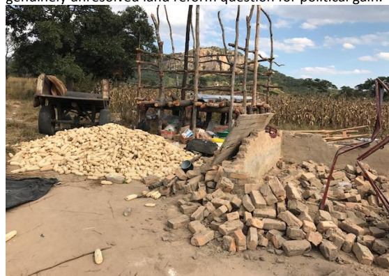
Fig 1.1 Demolitions Amidst Harvest Time
